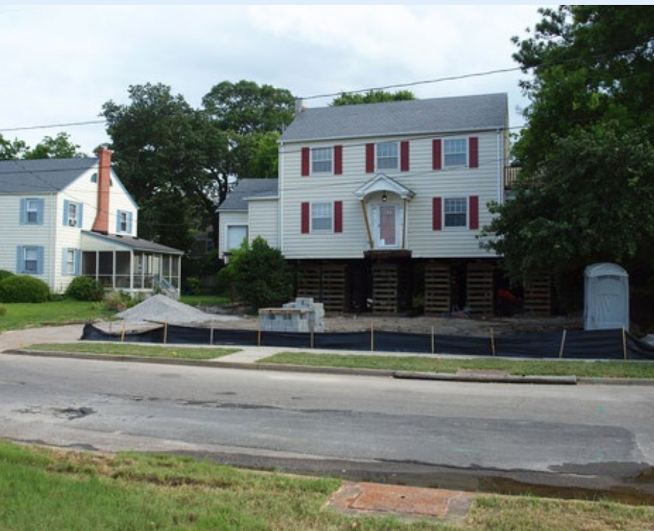
House being raised to reduce flood risk, Norfolk, Virginia
